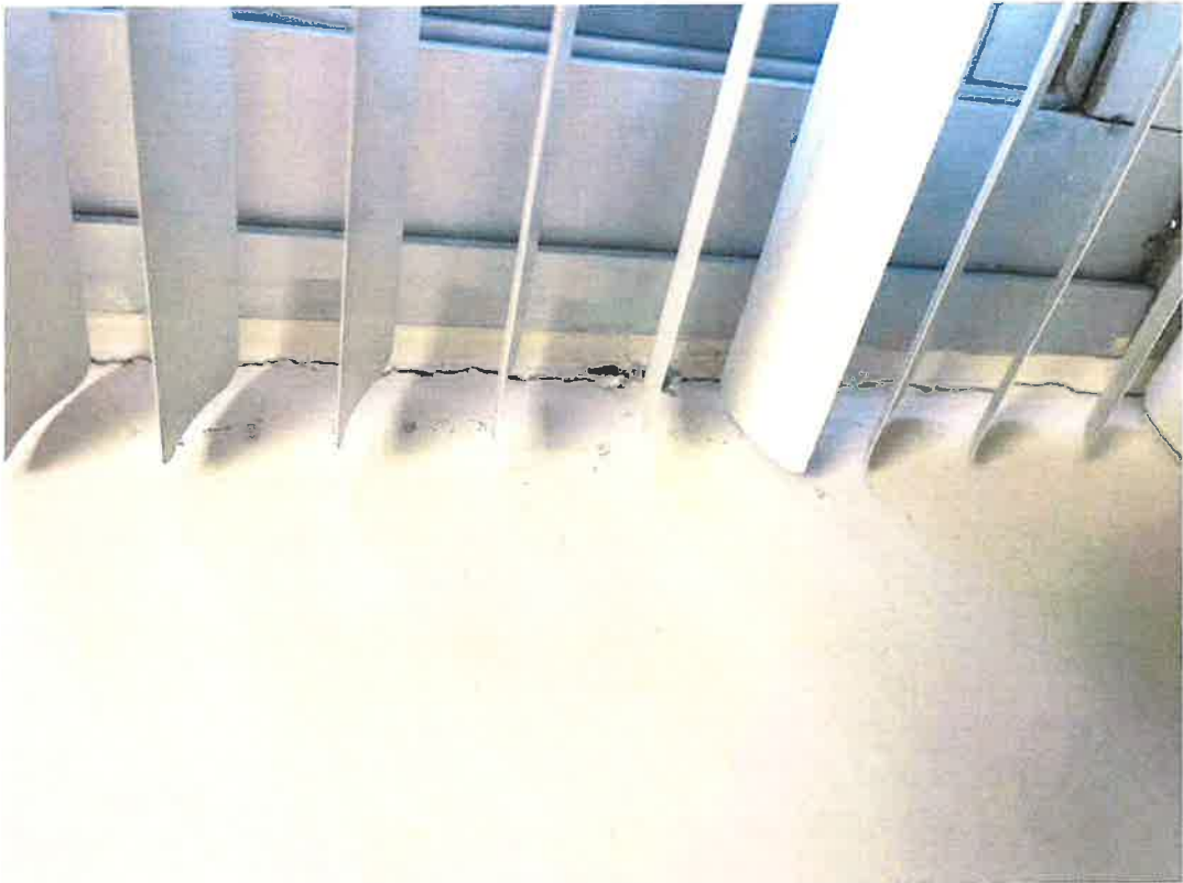
Upper Photo: M-02-Cementitious Panels
