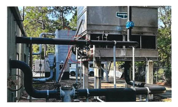
Answer #15: Confirmed the existing tower is piped incorrectly to support a second cooling tower. We will need to re-pipe in order to correct. Unfortunately, this will mean that the existing chiller will have some down time. This should be minimal if as much pipe is preinstalled and the final connections coordinated with college's schedule to avoid affecting the campus.
